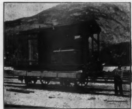
SAND BLAST CAR FOR RAIL BONDING.
