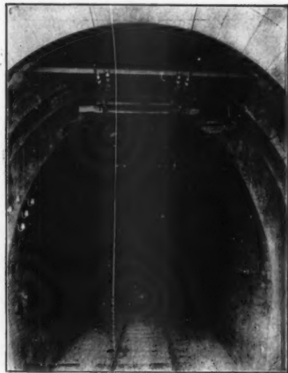
INTERIOR OF THE TUNNEL.
