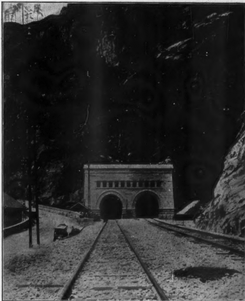
PORTAL ON THE ITALIAN SIDE AT DOMO D'OSSOLA. ENTRANCE TO BOTH TUNNELS CLOSE TOGETHER.
